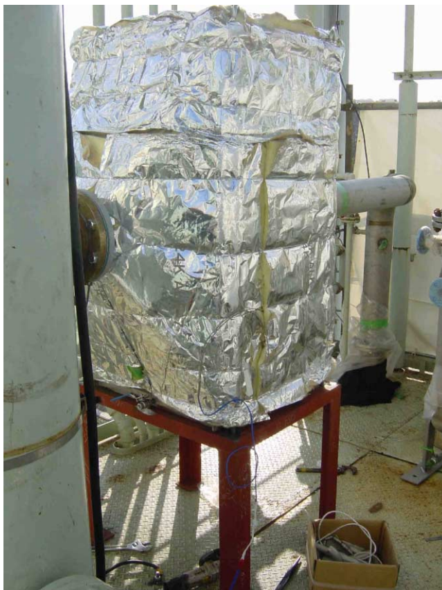
Figure 10: Test unit at the site.
