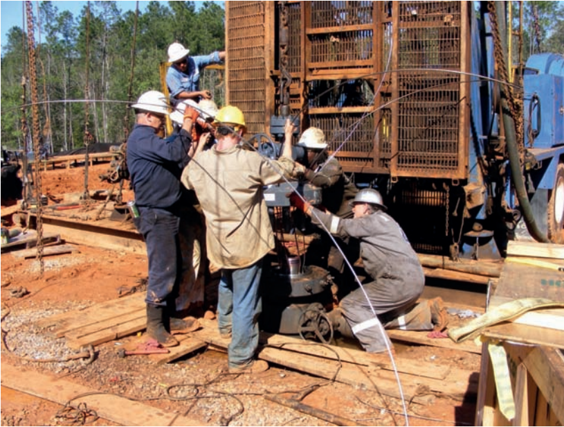
Figure 7. Feeding the control lines through the valve spool adapter after landing the tubing hanger.
