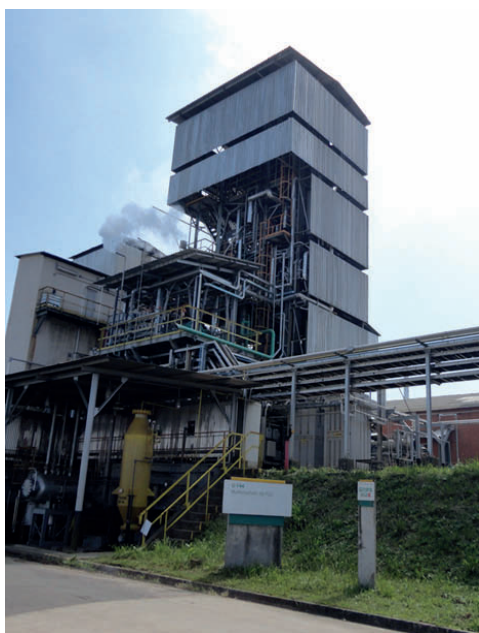
Figure 1. The FCC multipurpose test unit (courtesy of Petrobras).
