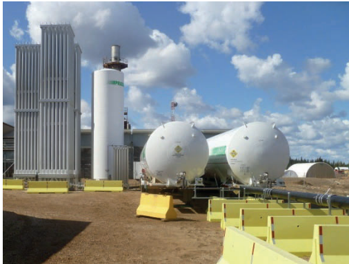
Figure 2. Oxygen storage and supply system (courtesy of Cenovus and Praxair).
