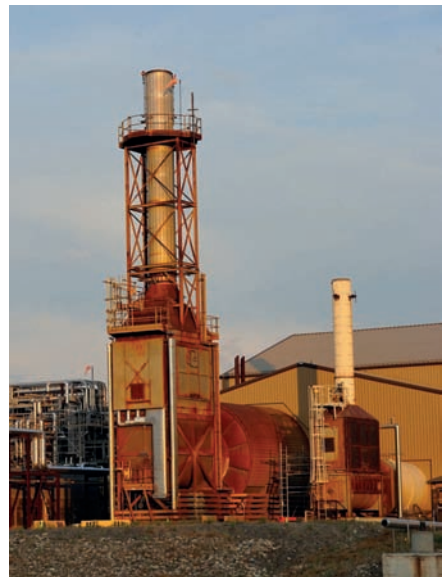
Figure 3. OTSG boiler for demo run in Christina Lake (courtesy of Cenovus Energy Inc.).
