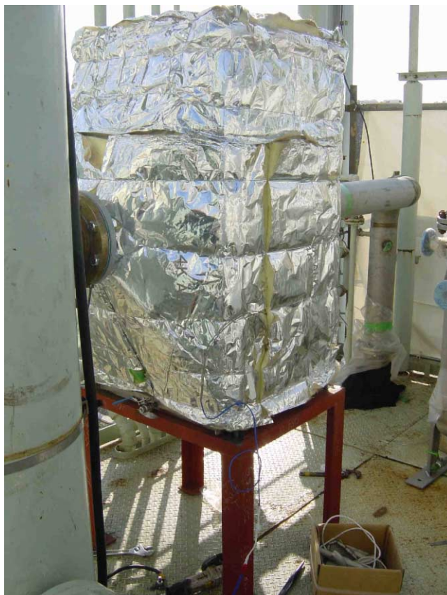
Figure 10: Test unit at the site.
