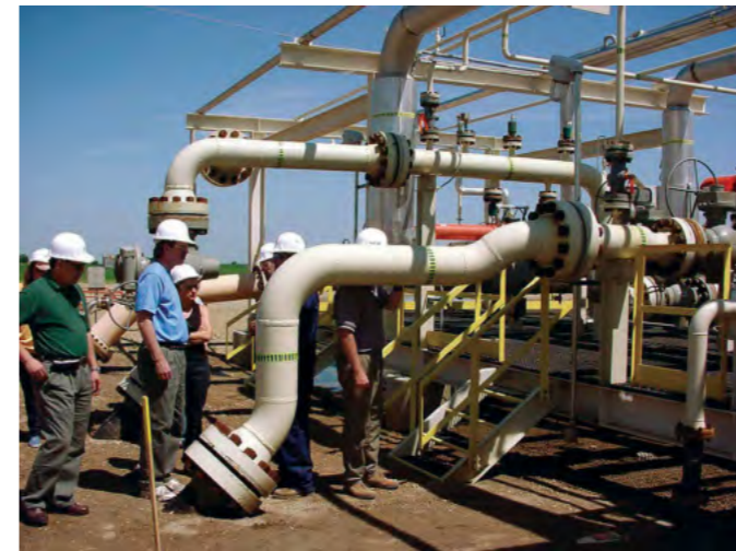
▲ CO 2 injection at Weyburn, Canada Image courtesy of Carbon Mitigation Initiative, Princeton University
